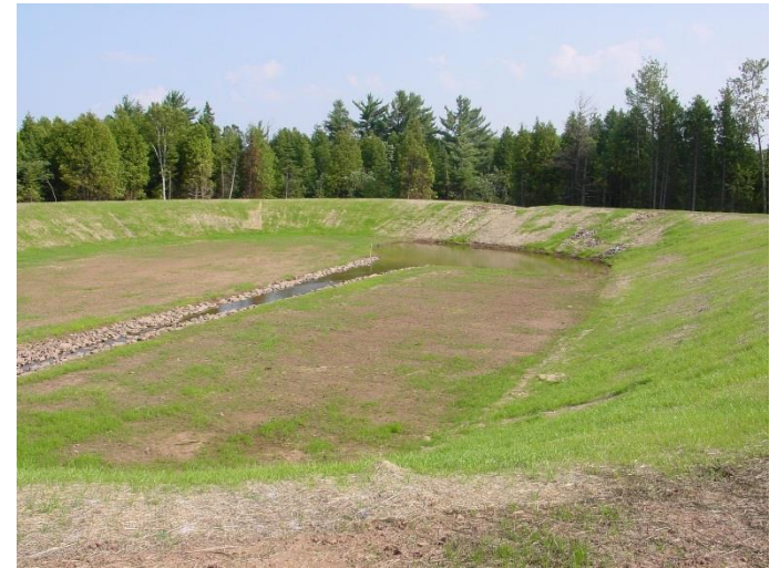
Photo – Dry detention pond
